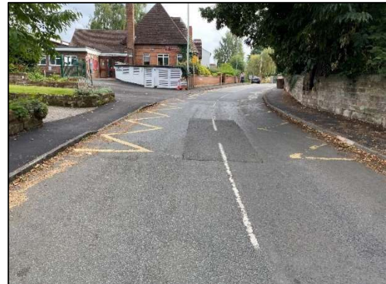
Figure 12: Bradford Road, Belbroughton
